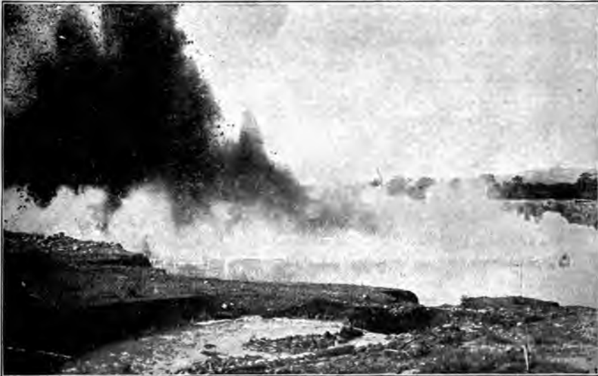
BLOWING UP THE DIKE AT MIRAFLORES WITH 40,000 POUNDS OF DYNAMITE, BEGINNING THE INFLOW OF WATER CONNECTING THE TWO OCEANS.
