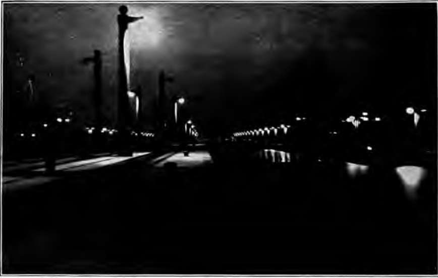
PEDRO MIGUEL LOCKS AT NIGHT, SHOWING ELECTRICAL ILLUMINATION OF THE CANAL.
