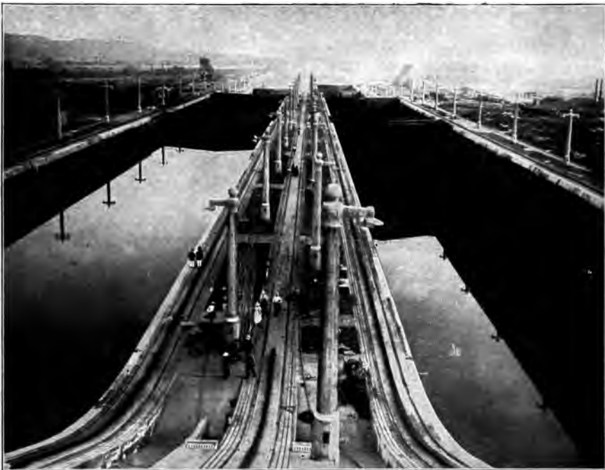
THE COMPLETED GATUN LOCKS, LOOKING NORTH TOWARD THE ATLANTIC ENTRANCE.
