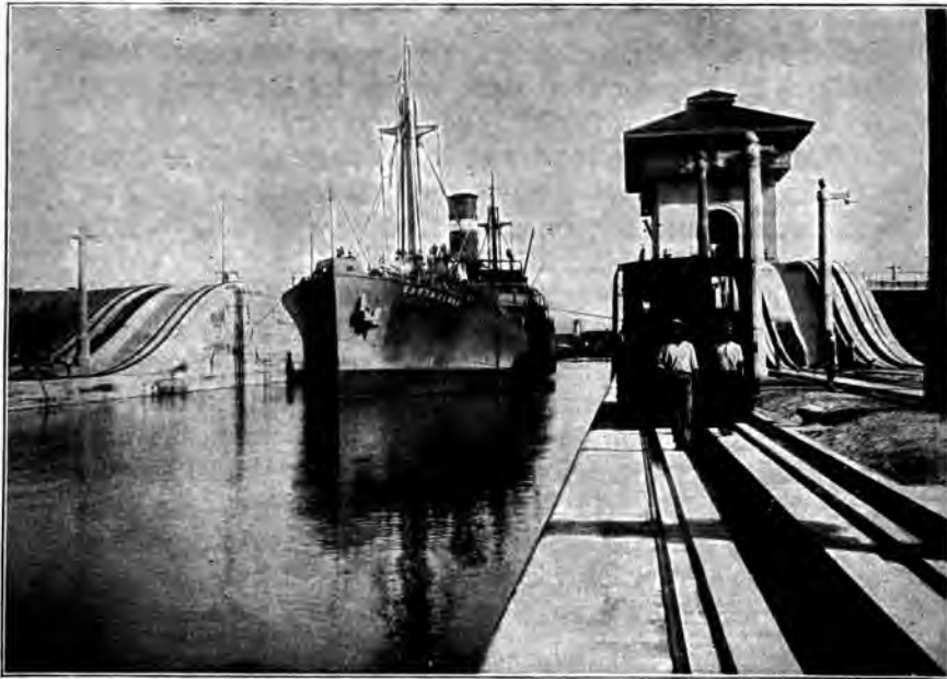
THE STEAMSHIP "SANTA CLARA" ENTERING MIRAFLORES LOCKS UNDER TOW OF ELECTRIC LOCOMOTIVES, JUNE 19, 1914.
