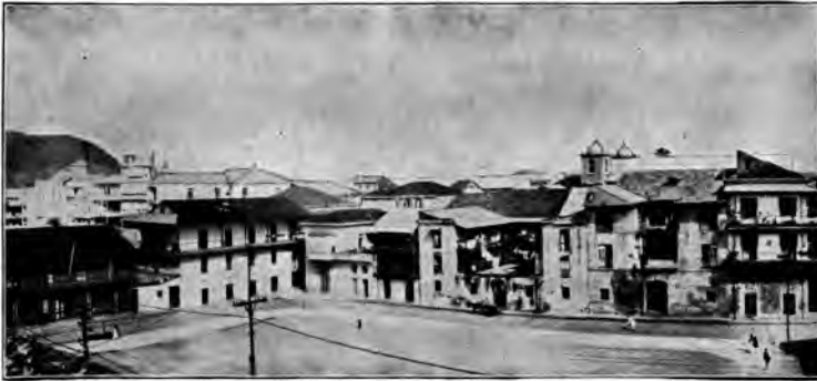
CORNER OF A PUBLIC SQUARE IN PANAMA CITY.
